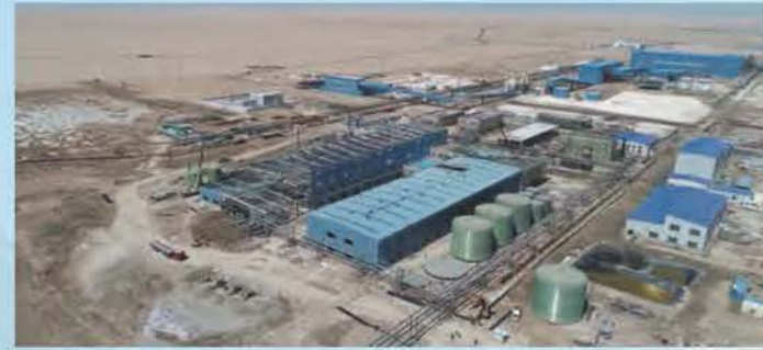
五矿盐湖项目 Project of Salt Lake for China Minmetals Corporation
