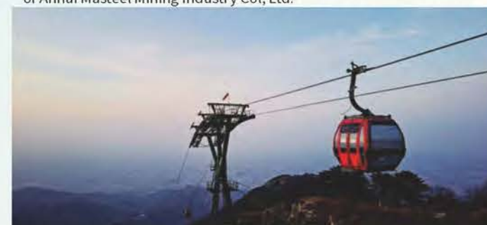
山东泰山中天门索道 Project of Zhongtianmen Ropeway on Mount Tai in Shandong Province
