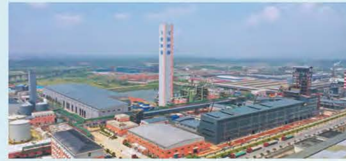
江西兴南危固废处置项目 Project of Hazardous Solid Waste Treatment for Jiangxi Xingnan Environmental Protection Technology Co., Ltd.
