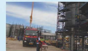
项目现场举行应急演练 Emergency drilling held on the project site
