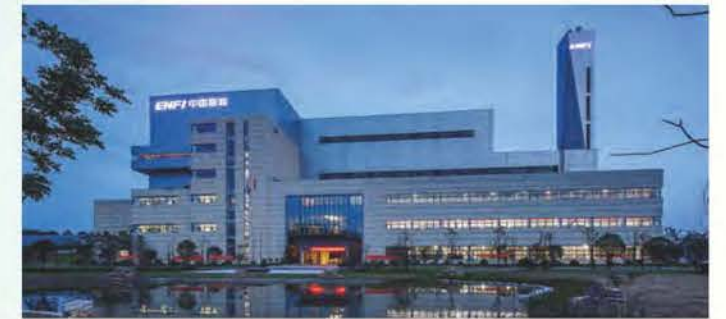
赣州市生活垃圾焚烧发电厂 Project of Domestic Waste Incineration Power Plant in Ganzhou City
