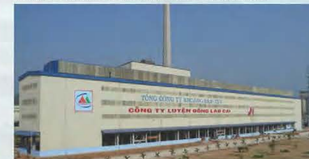
越南生权铜采选冶联合项目 Sin Quyen Copper Mining, Beneficiation and Smelting Complex, Vietnam
