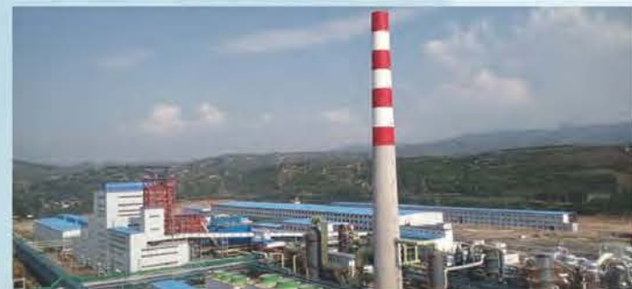
中原黄金项目 Project of Zhongyuan Gold Metallurgical Plant Co., Ltd.
